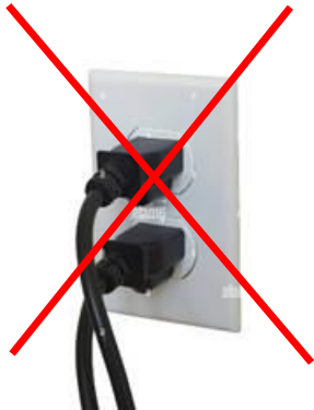
Two cords plugged into the same circuit is not recommended.
