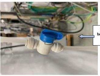
Hand valve. Connect building water supply or MPT adapter here
